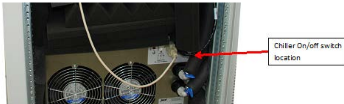
Figure 4.6 Chiller on/off switch Location
