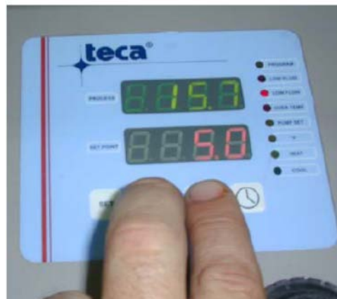
Figure 4.12 Pump Failed to Prime
